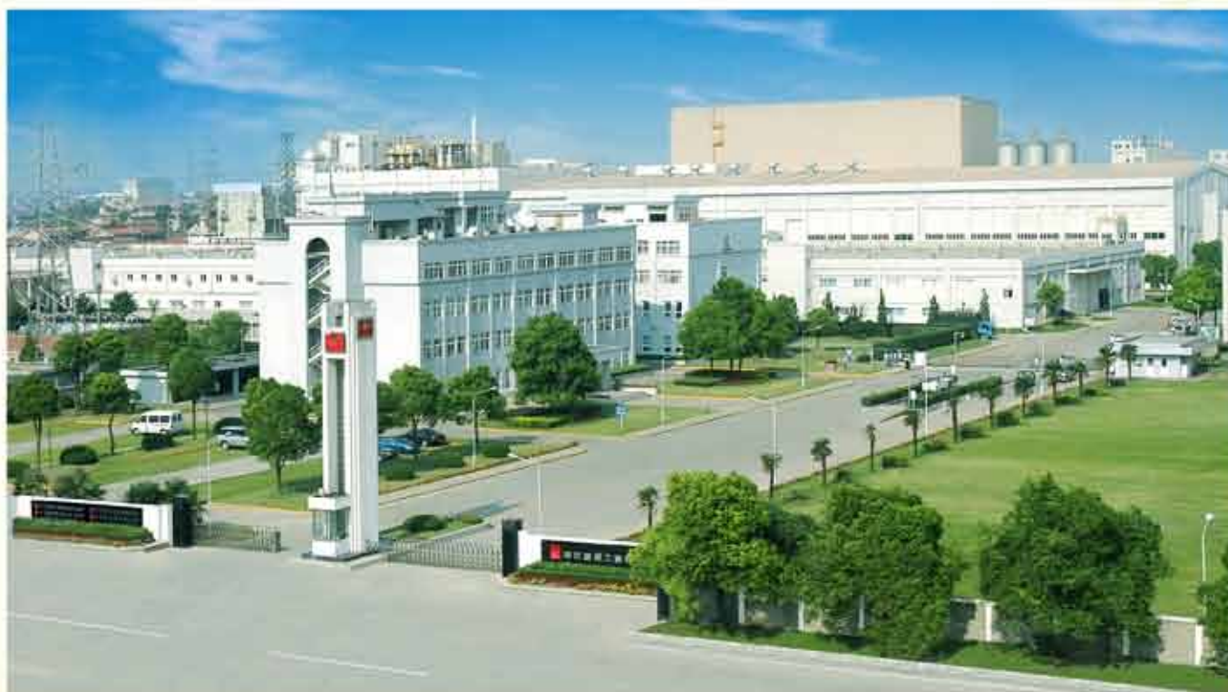
南通厂区 NANTONG Plant
